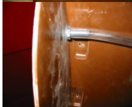
Picture 3 – vent outlet elbow on inside of box
