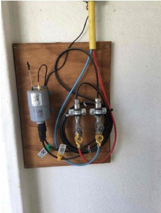
Typical pressure monitoring device installed in a vent stack cabinet
